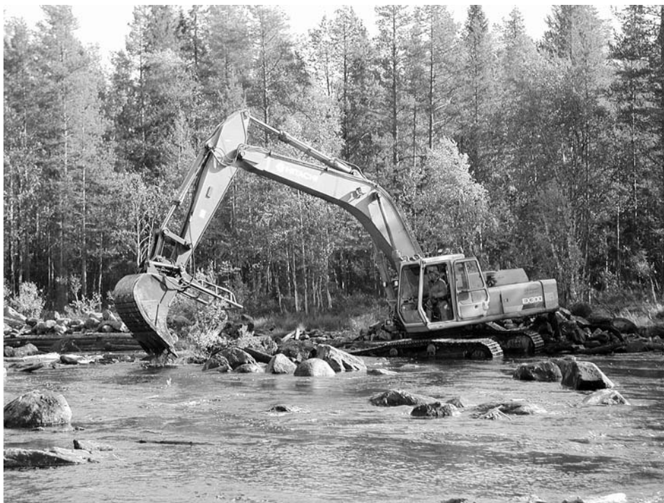
PLATE 1. Excavator removing a floatway structure previously separating a river channel from its riparian zone in northern Sweden. As the barrier is removed, boulders from the structure are relocated to the channel, thereby altering patterns of streamflow and fluvial disturbance. Such changes can enhance riparian biodiversity. Photo credit: C. Nilsson.
