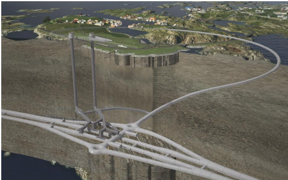
Image II: Overview of the Rogfast subsea road tunnel project, Stavanger, Norway. Source: Norwegian Public Roads Administration (40)
